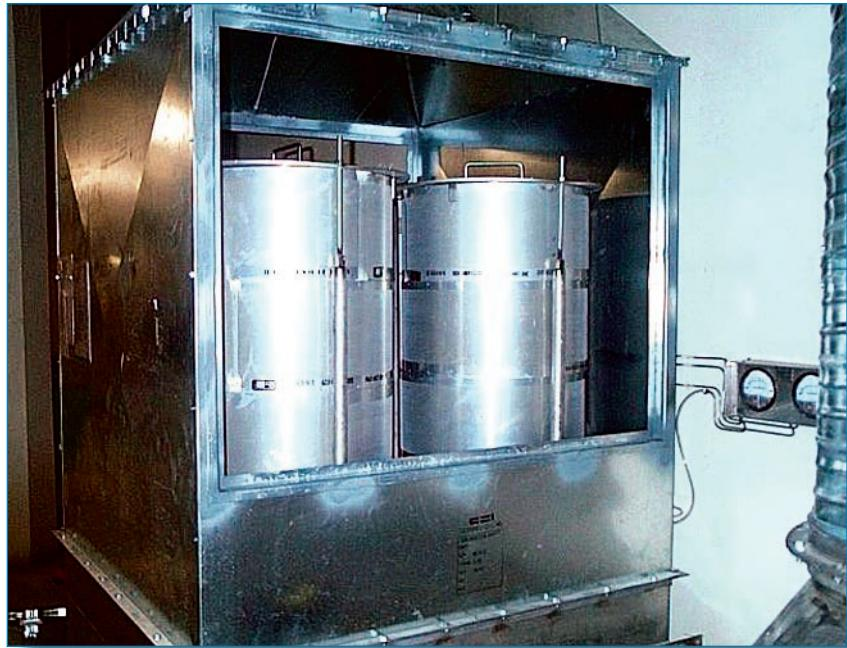
**Pre-heat Coil Module.** This module contains pre-filters, pre-heat coil, and an outside air damper. Pre-filters selected for the system are ASHRAE 25-35 percent pleated. The building in which this system is installed has chilled water and hot water service from a central plant.
